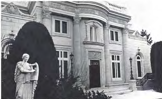
Front of the Belmar Mansion prior to demolition. Courtesy of Western History Dept., Denver Public Library
